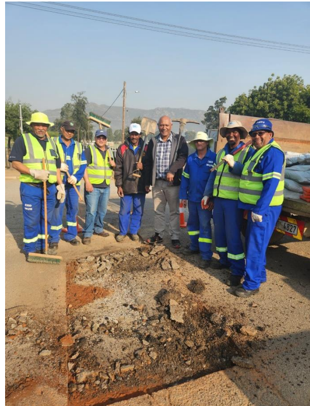
Mayor Ruben Richards joins pothole repairs teams in Citrusdal.
