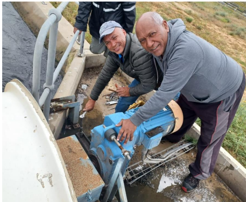
September 2023 – SUNDAY EMERGENCY BREAKDOWN - CE councillors (Andre Mouton [left] and Ruben Richards [right] fix pump at Municipal Sewerage Plant in Clanwilliam.
